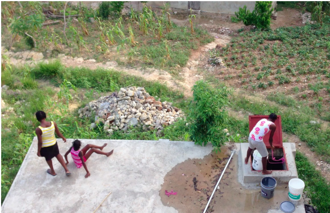
Women in Haiti draw water from an underground storage tank. The water is collected from rain runoff using pipes that direct the rain into the tank.
